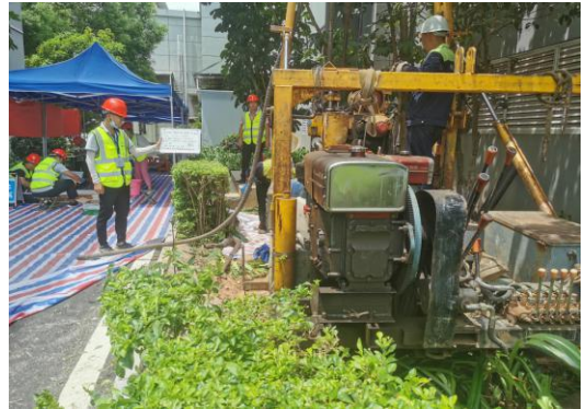
1A02-钻机类型、套管跟进
